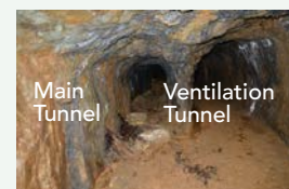
Mining tunnel Parallel tunnels for air circulation
