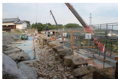
Repair of stonewalls of Komine-jo Castle Site (Shirakawa City, Fukushima Prefecture)
