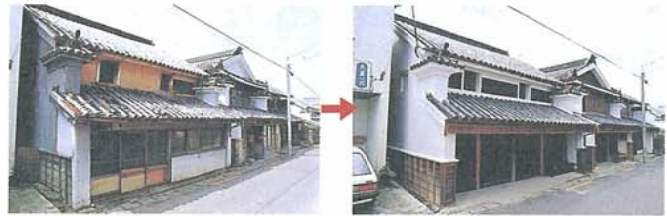
Repair of a historic building (Machiya) at Minamimachi, Waki-machi
