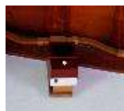
(光電分離式煙感知器)
