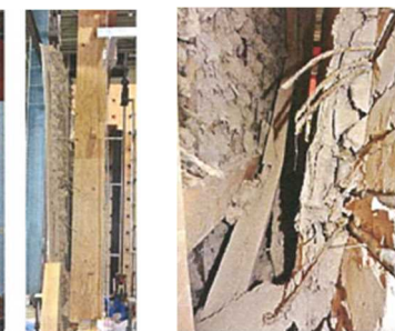
図14 筋違折損 (⑦)
