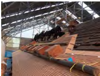
Photo 4-2 Re-roofing work on the main hall and worship hall of Hetsu-miya (2014)
