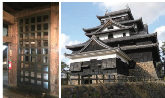
Seismic reinforcement for the keep, Matsue Castle, National Treasure
