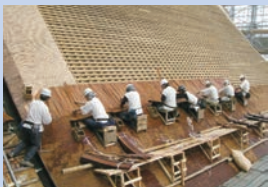
Roofing with Japanese cypress bark and wooden shingles
