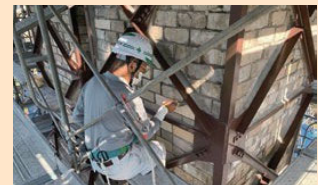
Repairing the bricks of the reverberatory furnace
