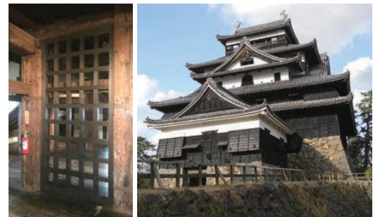
Seismic reinforcement for the keep, Matsue Castle, National Treasure
