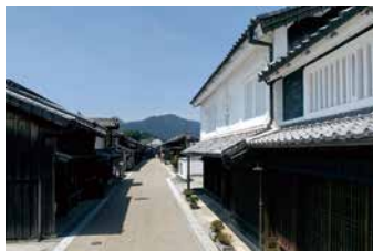
Important Preservation Districts for Groups of Traditional Buildings: Sekijuku, Kameyama City Photo: Courtesy of Kameyama City
