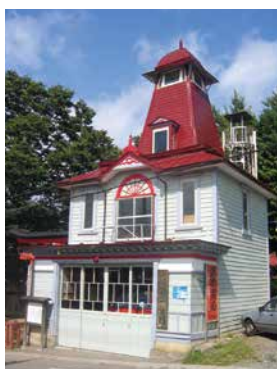
Stationing place No.1 of Gonohe Town Fire Company Important Cultural Property by Aomori Prefecture Photo: Courtesy of Aomori Prefectural Board of Education
