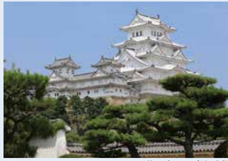
Photo Courtesy of Himeji City
