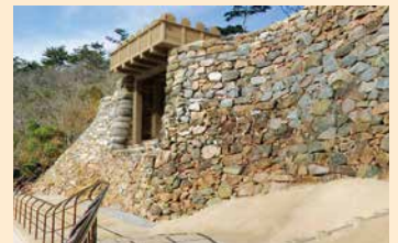
Restored stacks of stones and computer-generated gate
